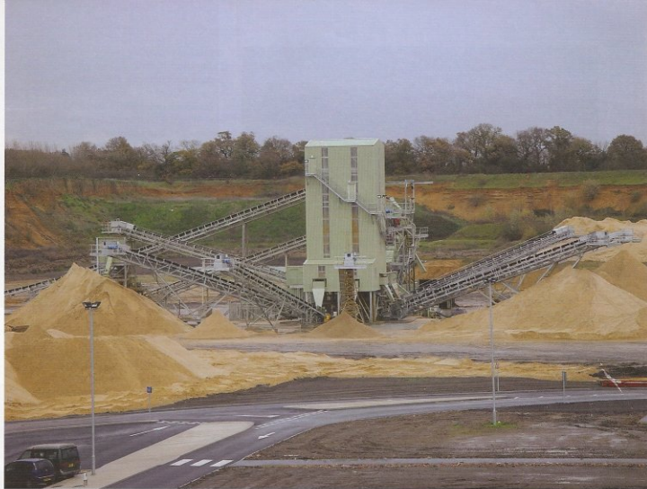
The new state-of-the-art sand and gravel plant at Tarmac's Colchester Quarry
