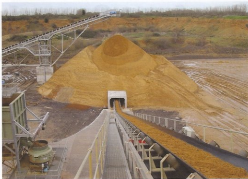
View showing the 4,000-tonne surge pile and recovery conveyor
