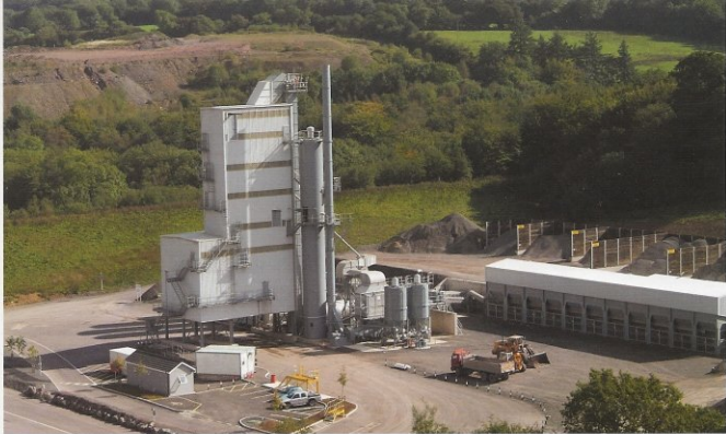
The new Benninghoven TBA240U asphalt plant at Moons Hill Quarry
