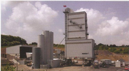
The plant includes a 360-tonne mixed-material storage section with direct lorry load-out
