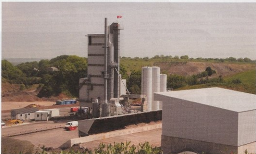
View of the 2,000 tonne structure and screening bunds
